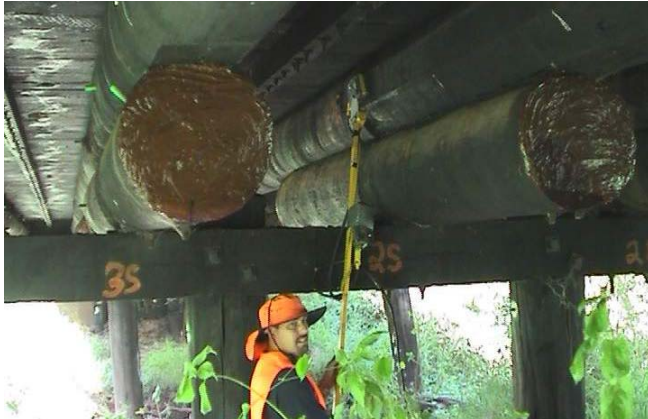
Figure 10 - GPR investigation of Redbank Creek (Crossing #3) Bridge
