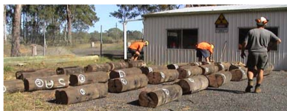
Figure 8 - Purga Creek Girders are cut up
