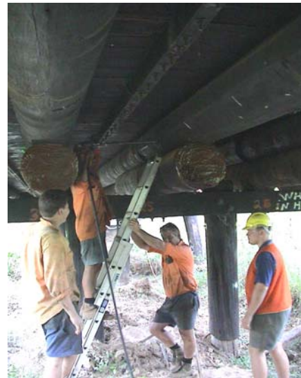
Figure 11 - Drilling investigation of Redbank Creek (Crossing #3) Bridge
