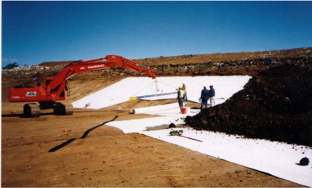
Figure 4: GCL base liner being installed and covered.
